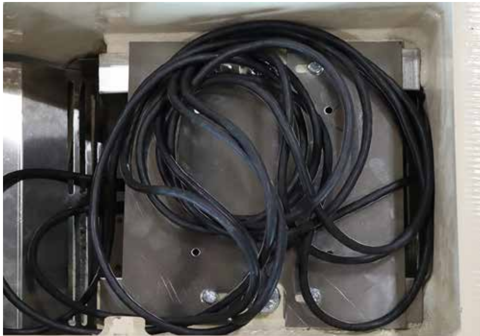
Figure No. 12 – Coil excess cable and place on the stainless steel cable tray.
