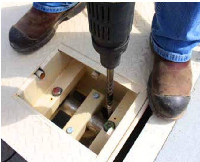
A 36-inch drill bit is required to clear the access opening when drilling the holes.
