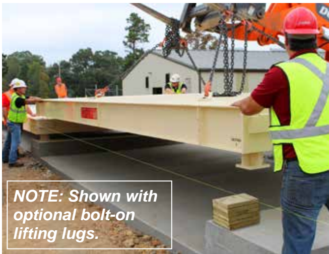
Lower second bridge onto wood blocks and support blocks of the first bridge.
