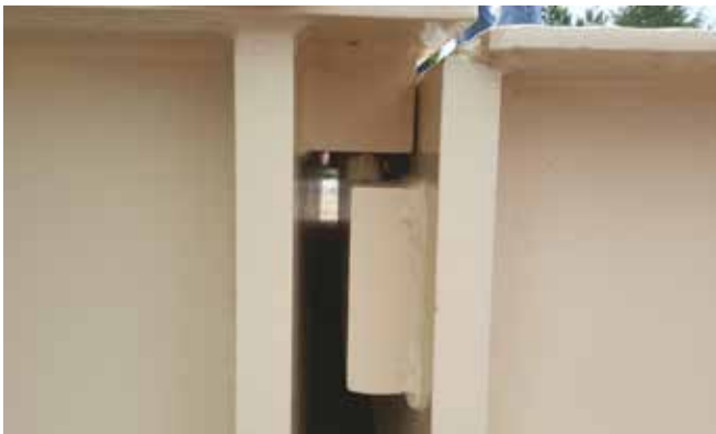
Second bridge receiver cup aligned with the first bridge support block.
