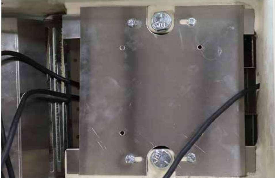
Figure No. 11 – Install the 1/4-20 x 3/4 in. hex head bolts to secure the load cell guards and stainless steel cable tray.
