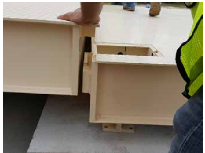
Align the second bridge receiver cups with the first bridge support blocks.
