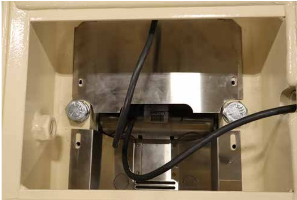
Figure No. 8 – First load cell guard cover installed and positioned over threaded holes.
