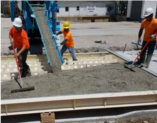
Placing the concrete.
