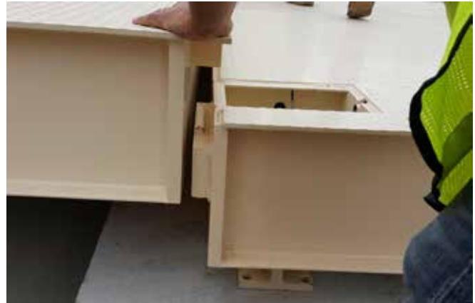
Align the second bridge receiver cup with the first bridge support block.
