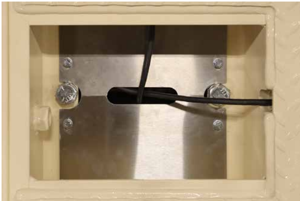
Figure No. 12 – View of completed Rodent Guard installation.
