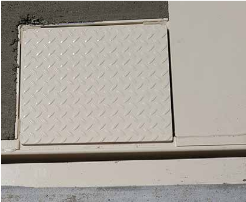
Figure No. 13 – Installed access plate on 8-inch beam concrete deck scale
