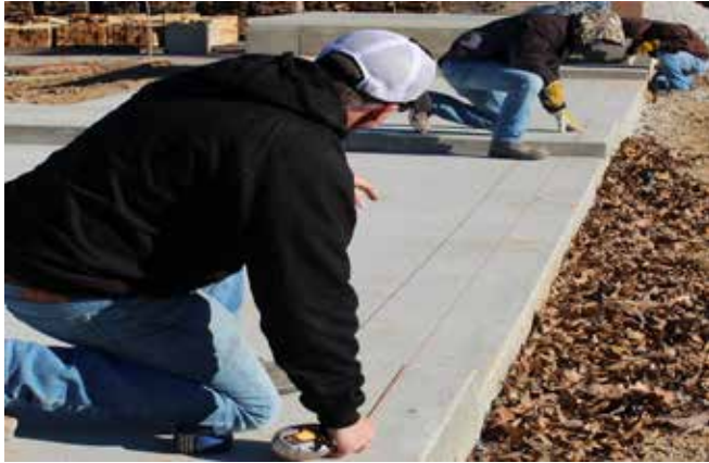
Snap a longitudinal chalk line on edge of piers per foundation drawing.
