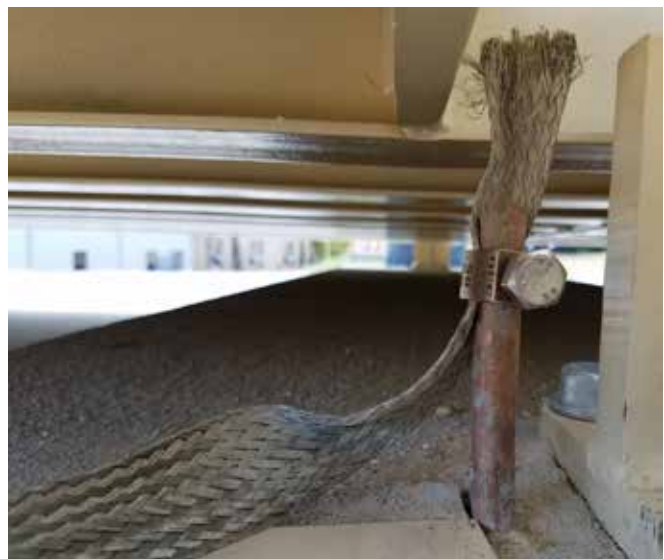
Ground Rod Connection
