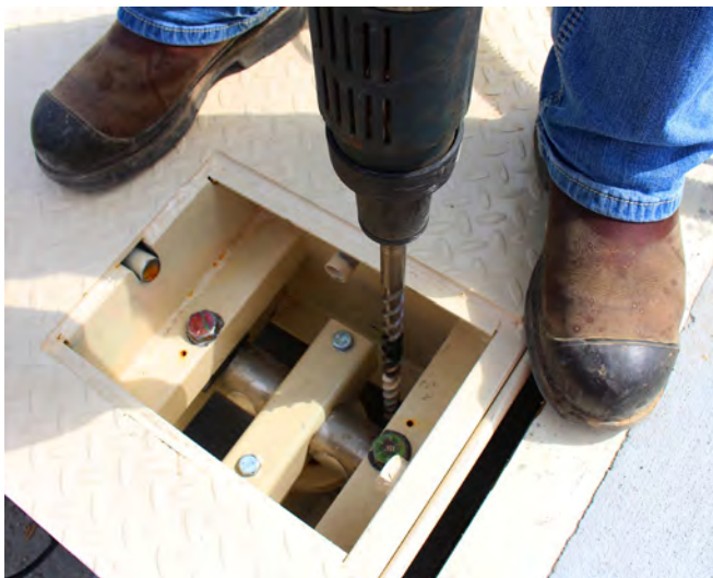
A 36-inch drill bit is required to clear the access opening when drilling the holes.
