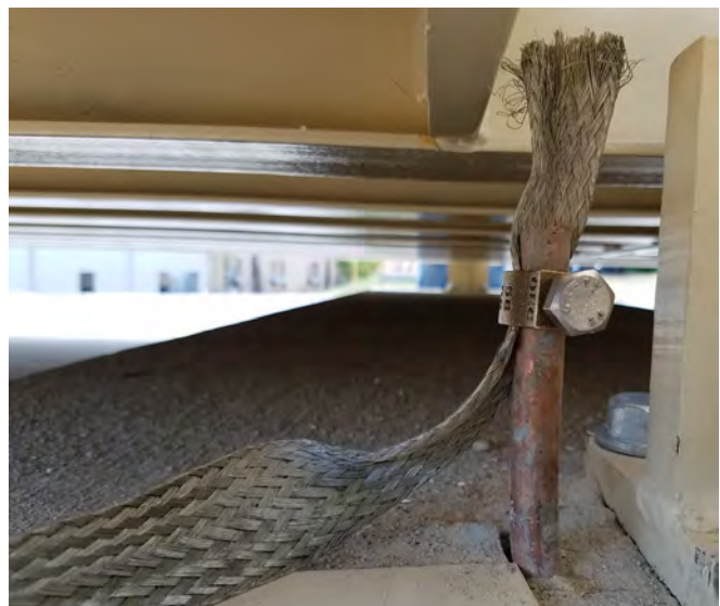
Ground Rod Connection
