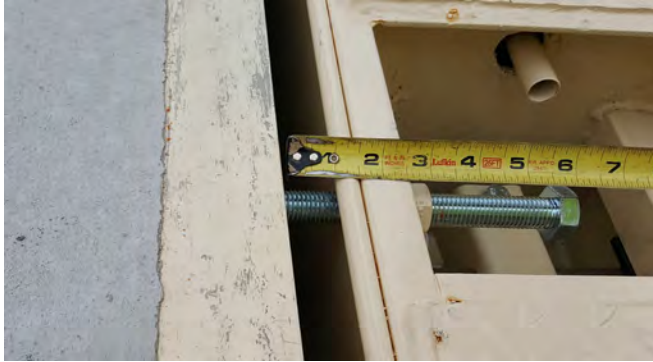
One-inch clearance is required from edge of the module to coping angle assembly.
