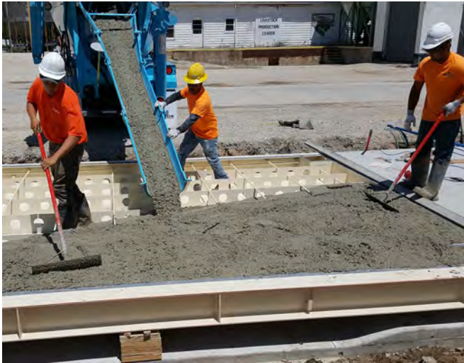
Placing the concrete.
