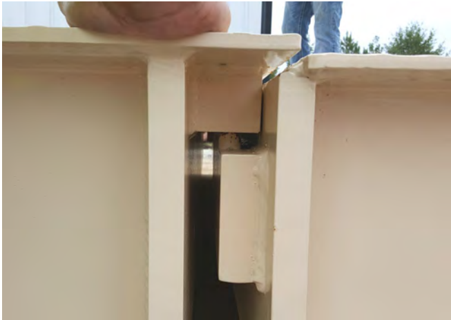
Second bridge receiver cup aligned with the first bridge support block.
