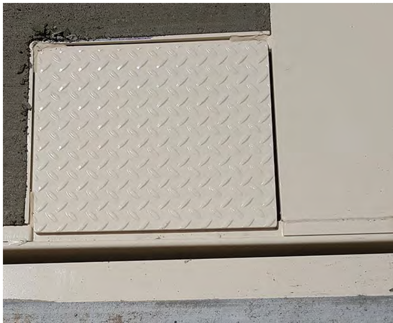
Figure No. 14 – Installed access plate on 10-inch beam concrete deck scale
