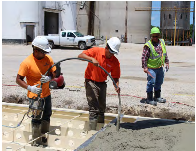
After the concrete has been placed, it should be vibrated.
