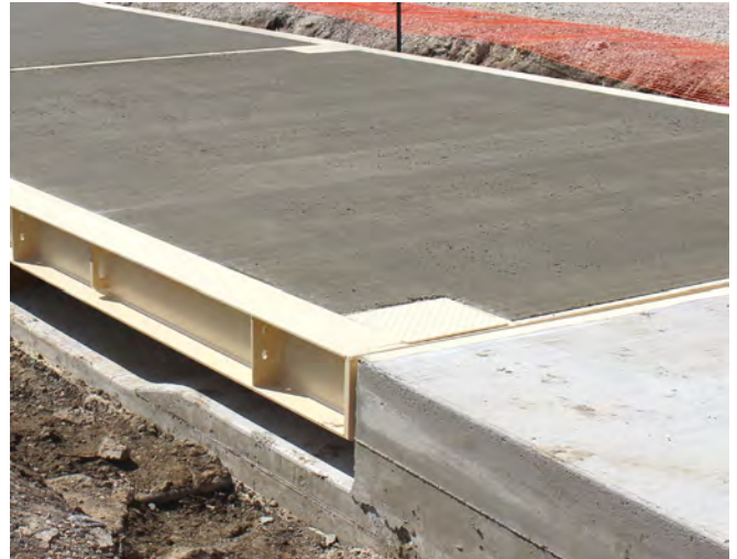
Apply a transverse texture to concrete with a wire broom (broom strokes perpendicular to the direction of traffic).
