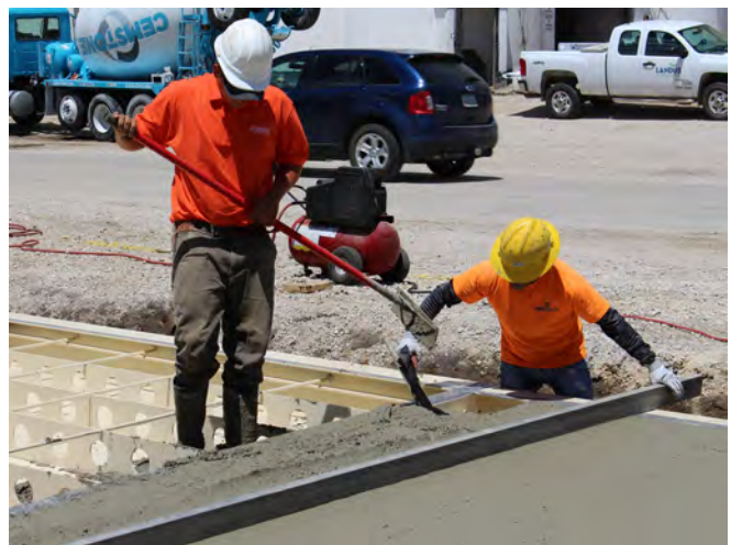
Keep a supply of concrete ahead of screed during screeding operation.
