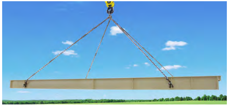
When being lifted by a crane, the additional brackets can be used to facilitate an equal balance of the bridge.
