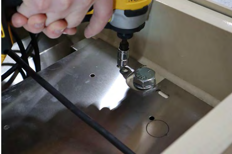
Figure No. 11 – Place the stainless steel cable tray under the cables in the load cell pocket.
