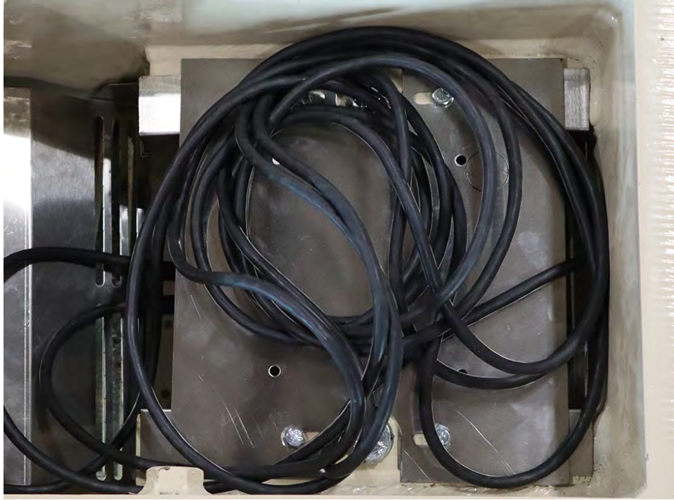
Figure No. 13 – Coil excess cable and place on the stainless steel cable tray.
