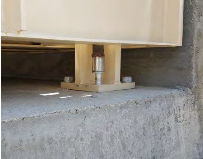
Insert anchor bolts and use a 1 1/8-inch socket and impact wrench to tighten.
