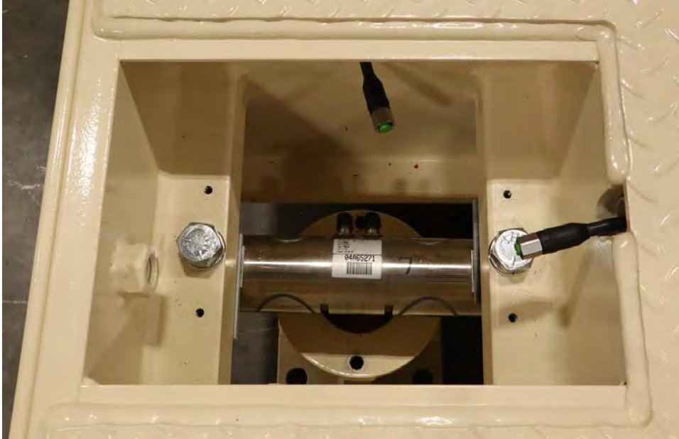
Figure No. 1 – With load cell cables installed, begin on the load cell connector side.
