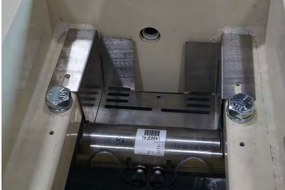
Figure No. 3 – Inner load cell guard installed and positioned over threaded holes.
