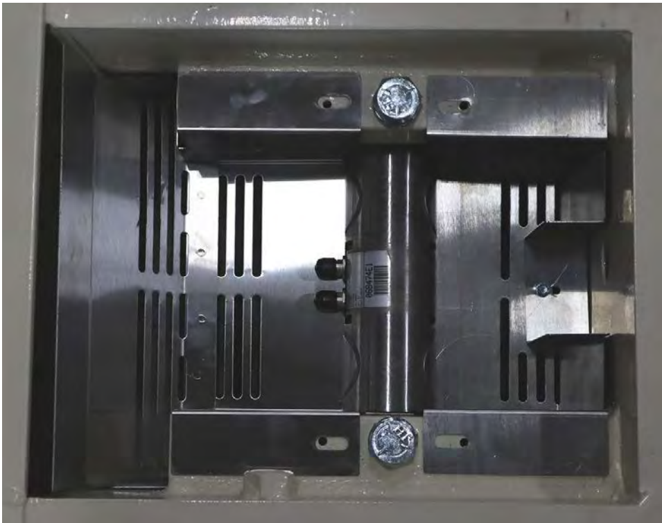
Figure No. 8 – View of both load cell guards and inner guard plate installed.
