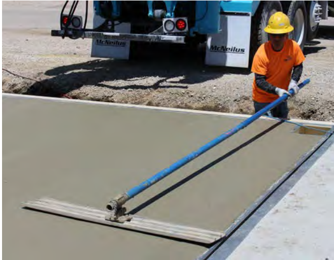
Before concrete becomes non-plastic, deck surface should be further finished to provide a uniform surface texture.
