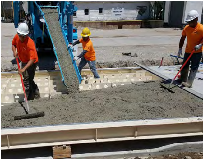
Placing the concrete.
