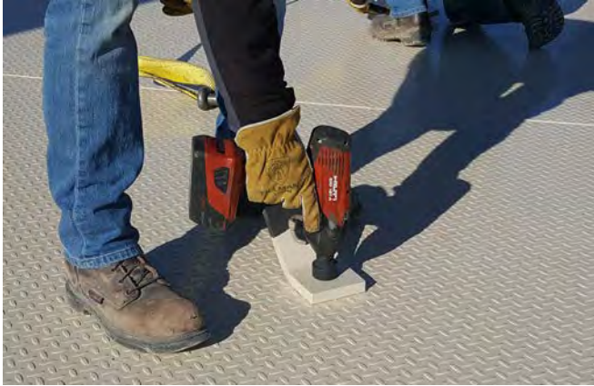
Remove the lifting lugs from the first bridge and install them on the second.
