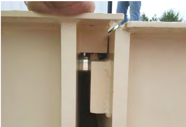
Second bridge receiver cup aligned with the first bridge support block.
