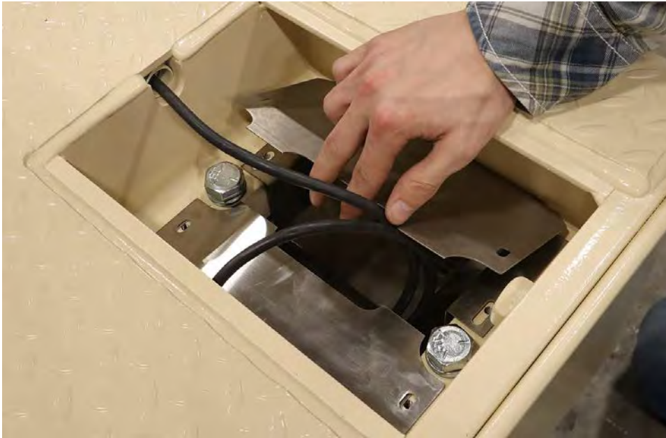
Figure No. 9 – Move cables to cut-out then place guard cover into load cell pocket.
