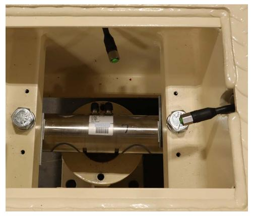
After installing the load cell cables into the scale conduit, position the cables so that only a small amount of the cable extends past the edge of the conduit.
