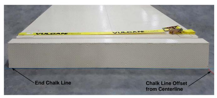
The bulkhead end should be on the end chalk line and the lower edge of the frame should align with the chalk line offset from the centerline.
