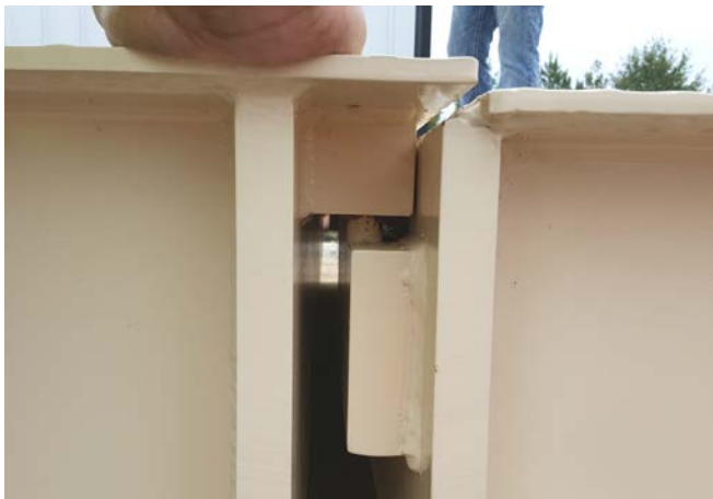
Align drop-in weighbridge receiver cups with end weighbridge support blocks.
