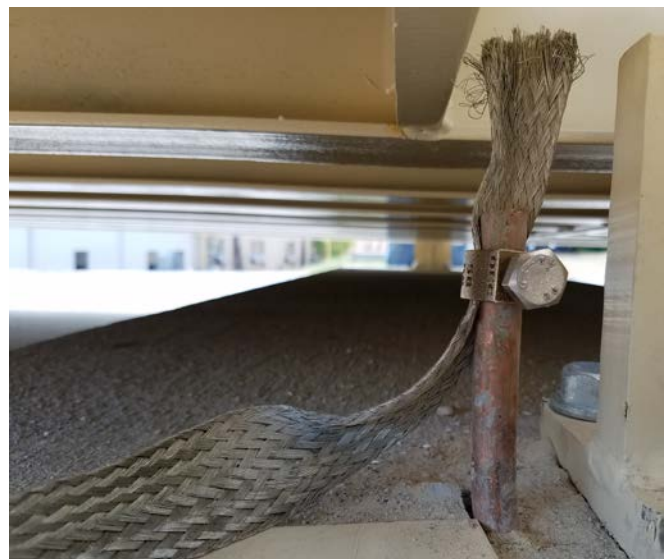
Ground Rod Connection
