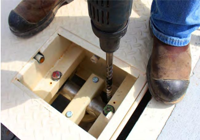
A 36-inch (90 cm) drill bit is required to clear the access opening when drilling the holes.
