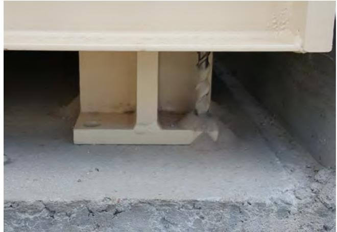
Drill 3/4 inch (19 mm) diameter holes 10 inches (25 cm) deep to install the anchor bolts.
