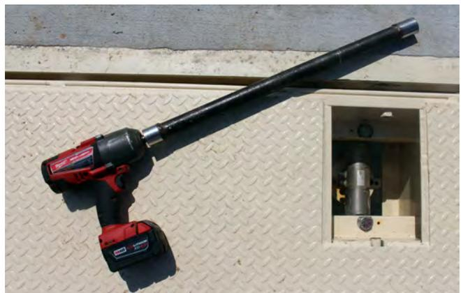
Insert the anchor bolts, and then use an impact wrench to tighten the anchor bolts.
