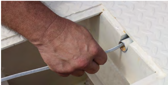
Insert load cell cable into the weighbridge conduit.
