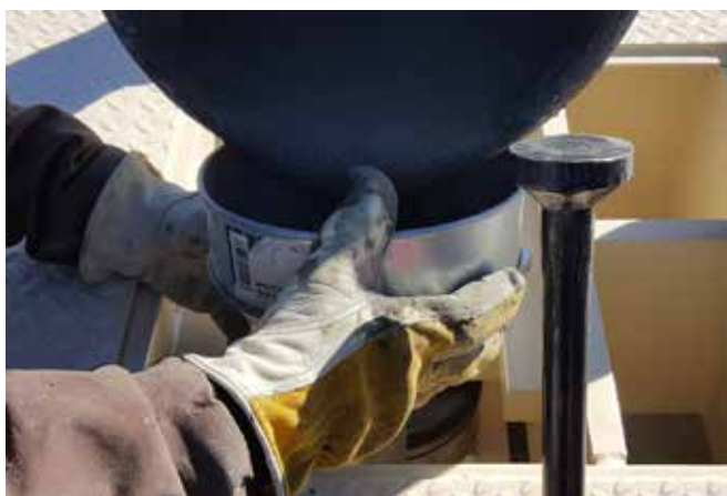
Pour grout into grout forms, allowing it to flow completely under the grout plate.
