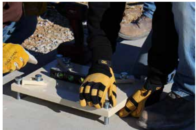
Place grout plate on the pier and ensure it is level in both directions.
