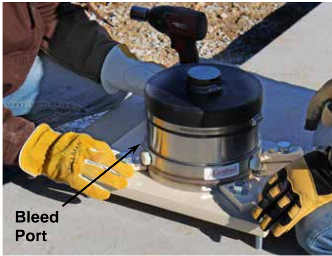
Place load cell on grout plate with bleed port pointing to outside of the scale.
