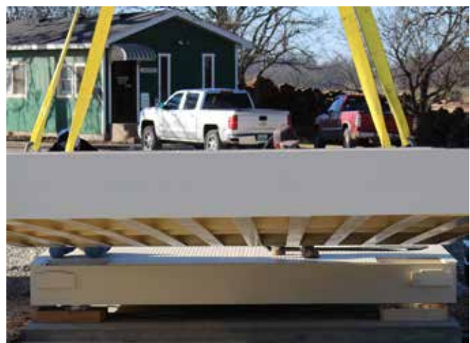
Align second bridge receiver cup with first bridge support block.
