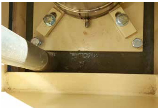
Make sure there are no voids under the grout plates.
