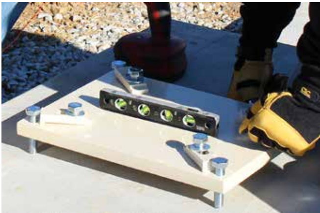
Place grout plate on the pier and ensure it is level in both directions.
