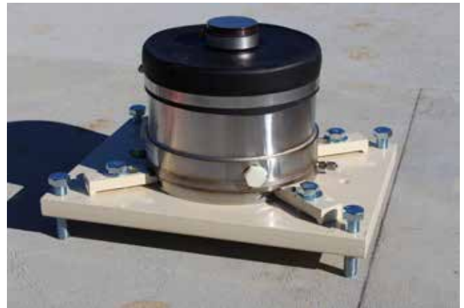
Check to make sure the grout plate is still correctly aligned on the pier.
