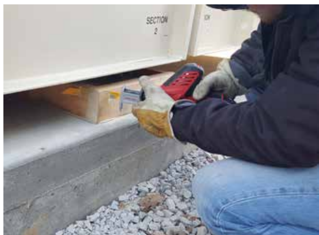
Allow grout to dry overnight before removing forms and loading scale.
