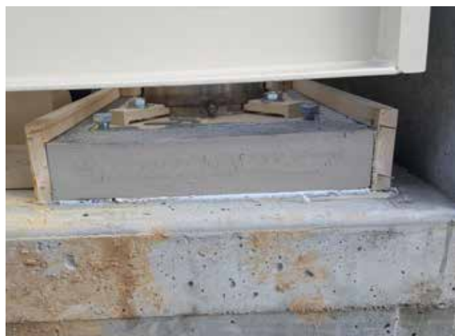
Allow grout to dry overnight before removing forms and loading scale.
