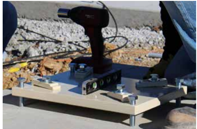
Place grout plate on the pier and ensure it is level in both directions.
