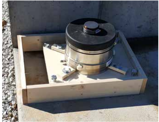
Grout forms in place around grout plate and load cell assembly.
