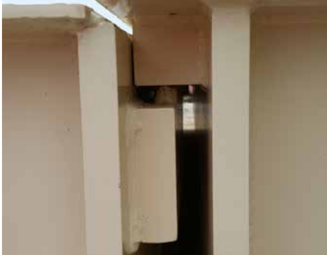
Bridge receiver cup aligned with bridge support block.
