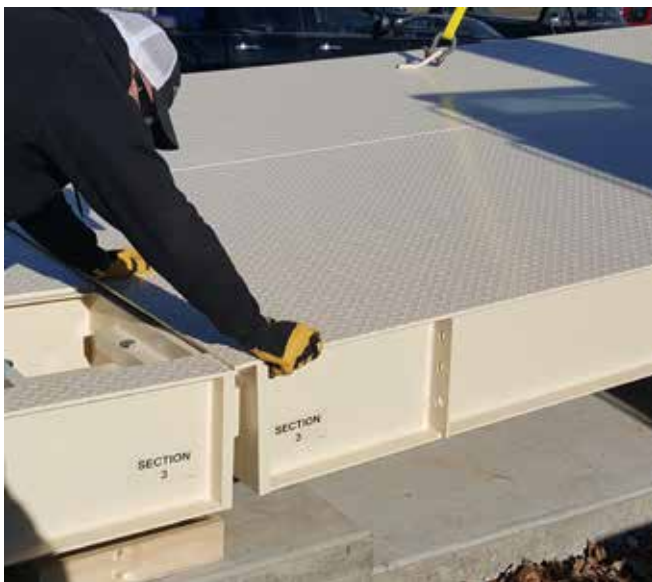
Lower bridge module receiver cup onto previous bridge module support block.
