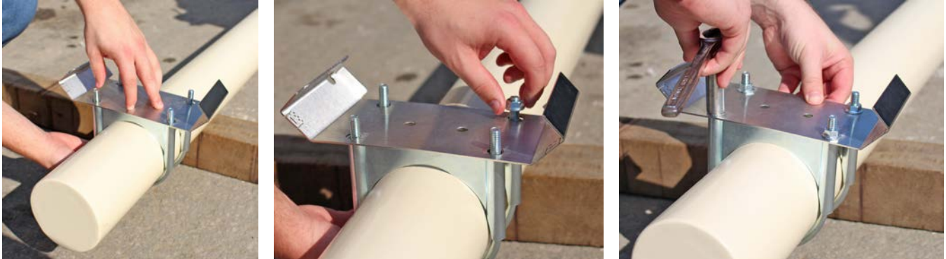
Figure No. 7 – Install Pole Bracket on Pole
