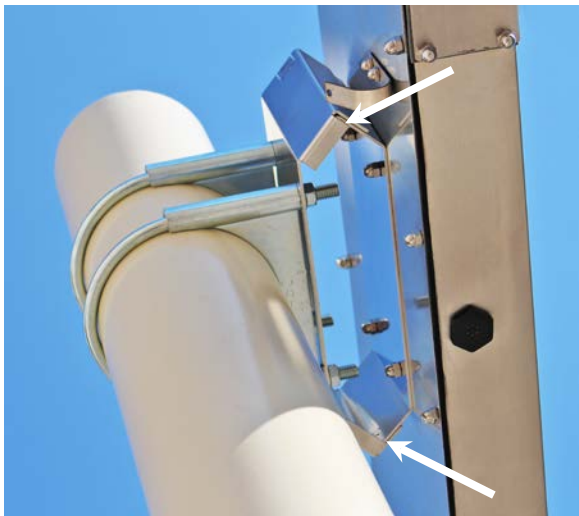
Figure No. 10 Ensure Brackets are Together
