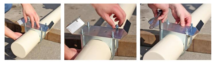
**IMPORTANT!** Visually check both sides of the pole to ensure the U-bolts are completely tightened against the pole.
