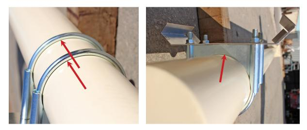
**3.** With the pole installed, align the bracket on the back of the SB600 with the bracket on the pole. Lower the SB600 until the top of the two brackets are flush with each other.
