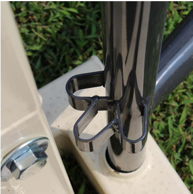
Lower stops on Gathering Panel tube.
