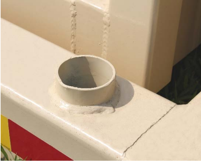
Frame opening for Gathering Panel tube.
