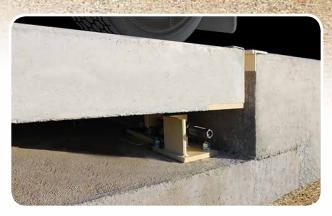
Clearance underneath the Harvester® truck scale's weighbridge is 7.5 inches from the top of the pier to the bottom of the deck which allows plenty of room for washouts and easy access to the load cells.
