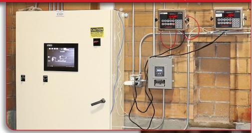
The end result is RMS' milling system providing an efficient, fast, and exact process for milling grain in brewery operations. "Our milling systems are designed to help breweries like Remedy expand their business and easily meet their production numbers. Cardinal Scale's THBC electronic load cell kits and 210 indicators are a big part of that system," says Riley Aadland, Applications Engineer for RMS Roller Grinder.
