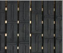
X-Lug flooring with open spacing between floor boards to avoid sewage congestion.
